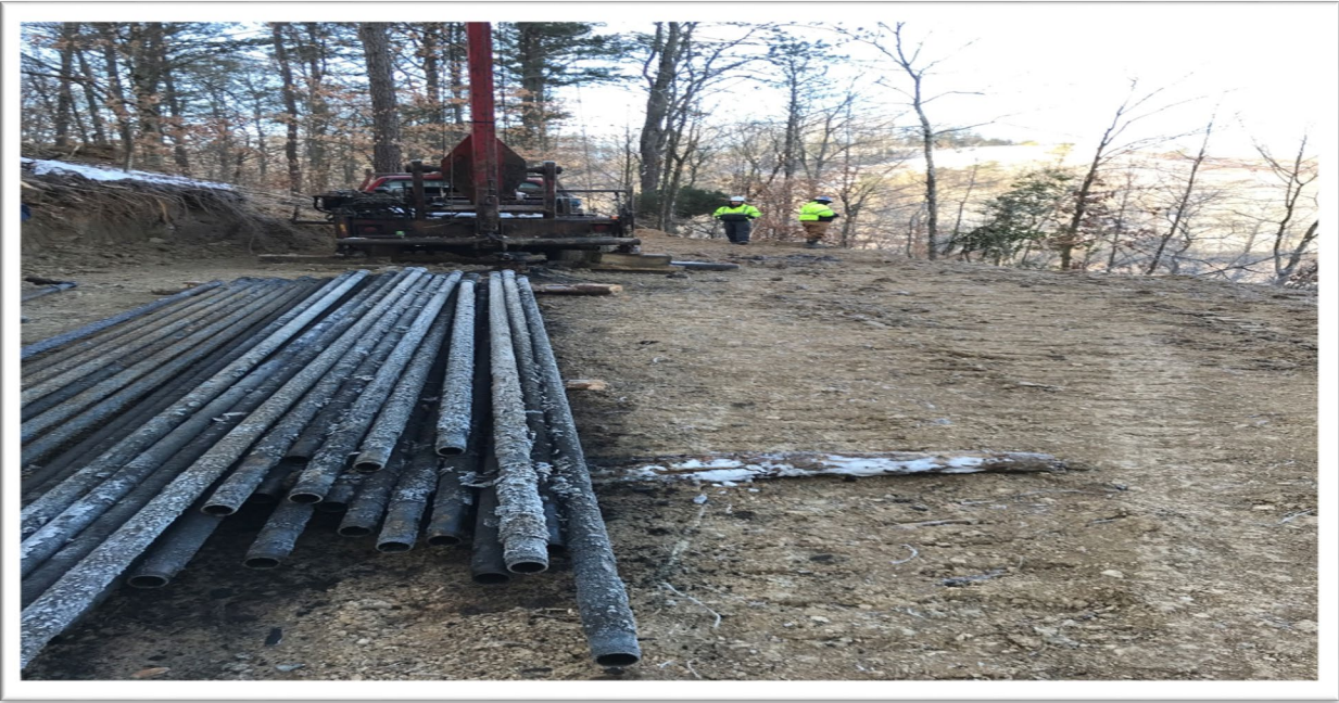
Figure 9: RN Sparks Crude Oil Spill, emergency well plugging activities.
