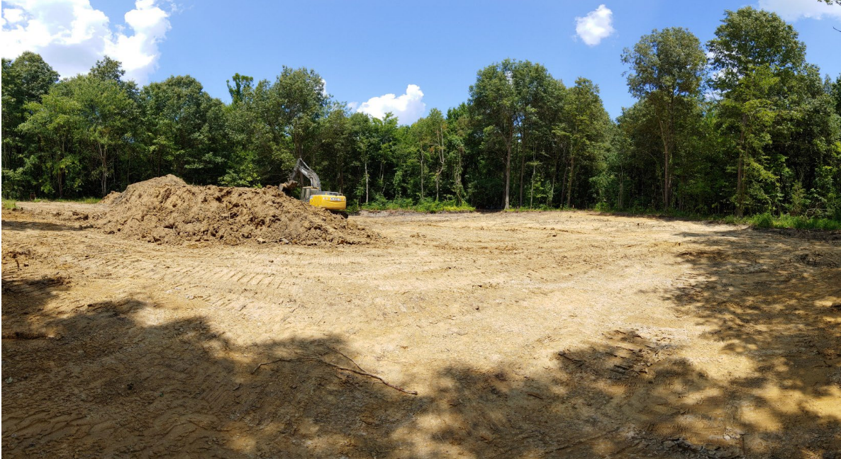
Figure 19: July 2021 – Looking north across the northern portion of the main removal area after the impacted spoil was stockpiled for disposal.
