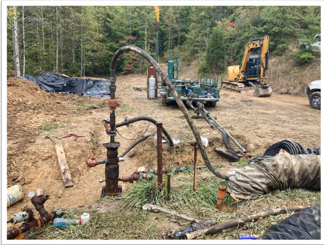
Figure 7: L&N Leaking H2S Gas Well, flaring of well prior to emergency plugging.
