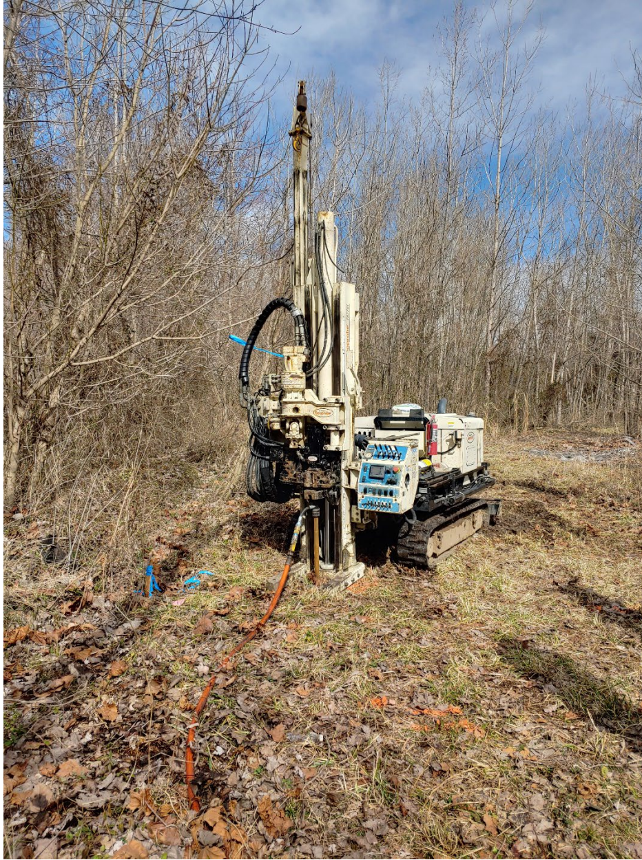
Figure 13: View of the equipment used during the injection process
